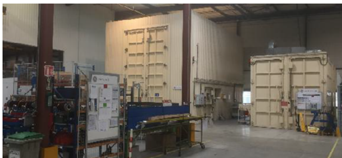
High-voltage dielectric, electronic and mechanical testing capabilities at GE Vernova's GCB Service Worldwide Center of Excellence.
