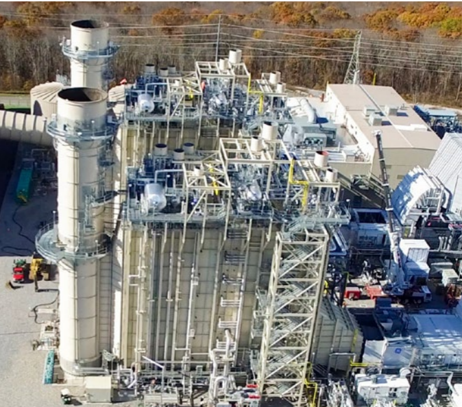
Towantic Power Plant, 7HA.01 2×1 805 MW multi-shaft combined cycle power plant, CPV Towantic Energy Center, Oxford, CT.
