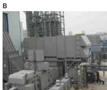
FIGURE 13: A: Frame 9E.03 operating on steel mill gases at a plant in China; B: LM2500+ operating on high H 2 coke oven gas
