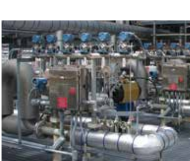
FIGURE 12: Hydrogen/natural gas blending system
