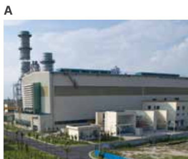
FIGURE 13: A: Frame 9E.03 operating on steel mill gases at a plant in China; B: LM2500+ operating on high H 2 coke oven gas
