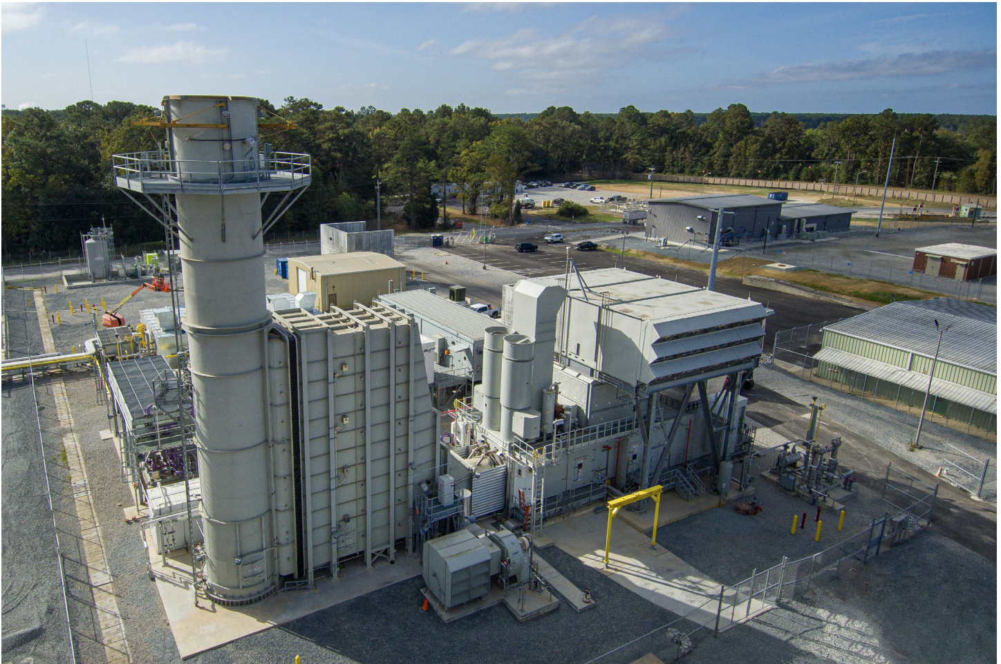
Figure 1: LM6000* gas turbine generator constructed with synchronous condensing capability
