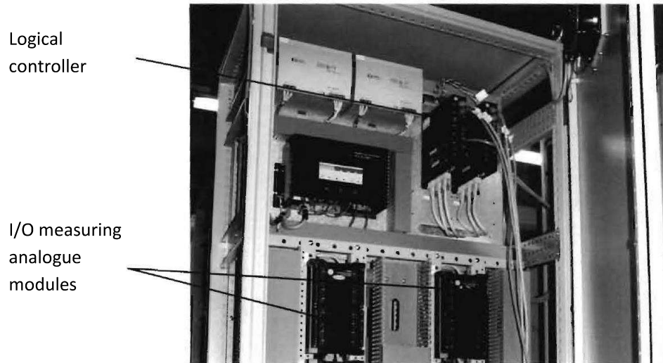
Figure 3 MCC components
