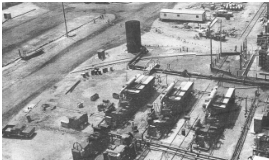
Figure 1. Belle River air-blow compressor layout. Note areas barricaded during blows.
