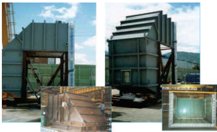
Figure 35. Frame 7E plenum during installation.
