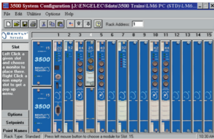
Bently Nevada Vibration System Display
