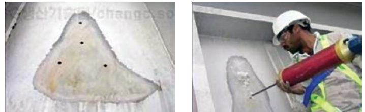
Figure 4: Re-fill insulation
