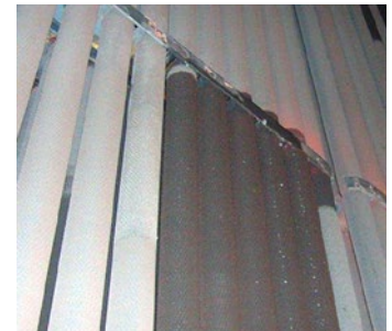
Figure 2: Leaking tubes from damaged restraints
