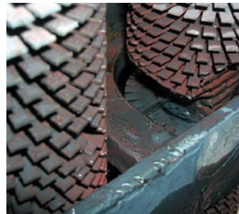
Figure 2: Leaking tubes from damaged restraints
