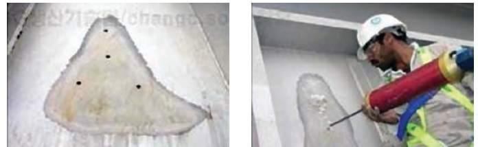
Figure 4: Re-Fill Insulation
