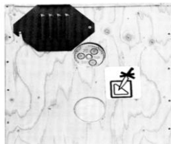
Figure 34: Open inspection opening with indicator
