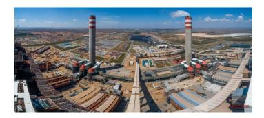
In 2018 Kusile's Wet Flue Gas Desulphurization (WFGD) plant, the first of its kind installed on the continent, exceeded its performance test by achieving a 93% removal efficiency rate for SO<sub>2</sub>.
