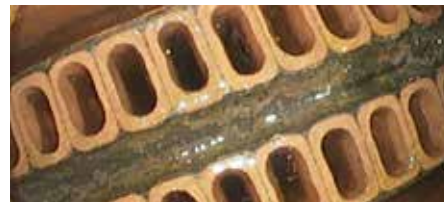
Water box treated
