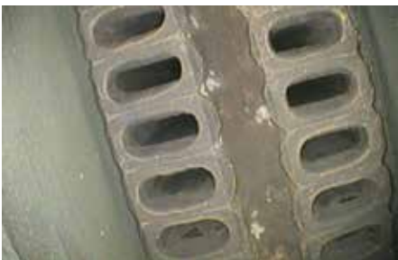
Water box being processed
