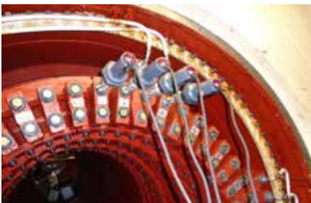
Water box being processed
