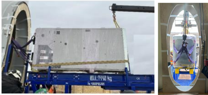
Figure 8 may illustrate cabinet movement from the sleigh into the tower.
