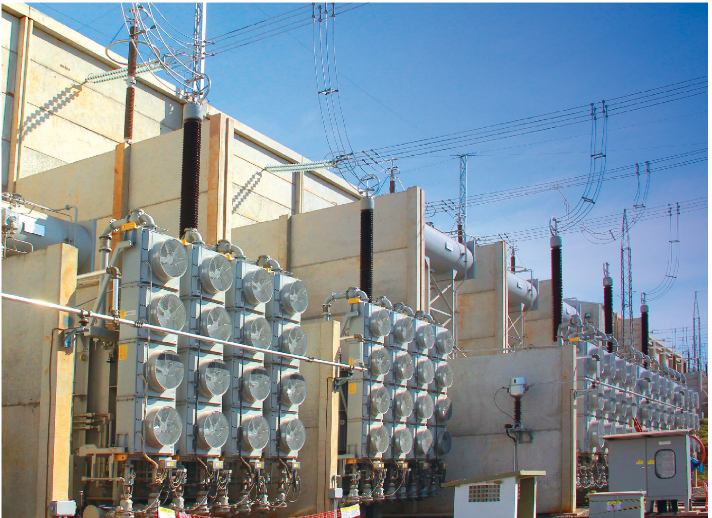
Converter Transformers
