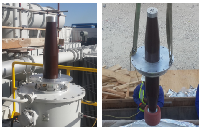
Fig. 4: Eyebolt for lifting
