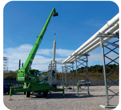
6. Installation of a 420 kV GIL in Kintore, Scotland
