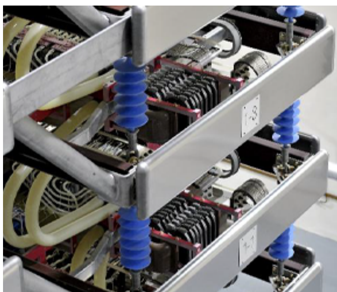
H400 thyristor valves
