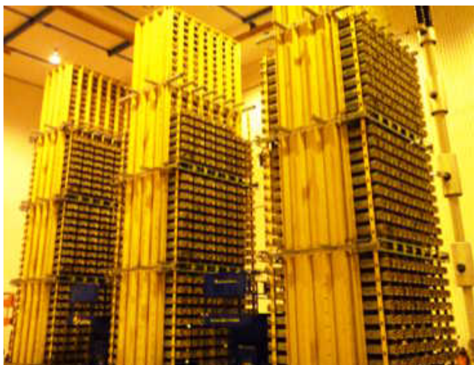
During the refurbishment
