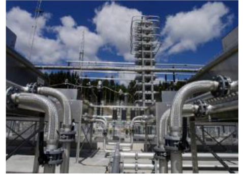
Outdoor valve cooling system
