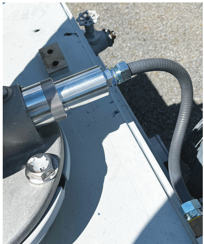
Sensor Test Tap Adaptor
