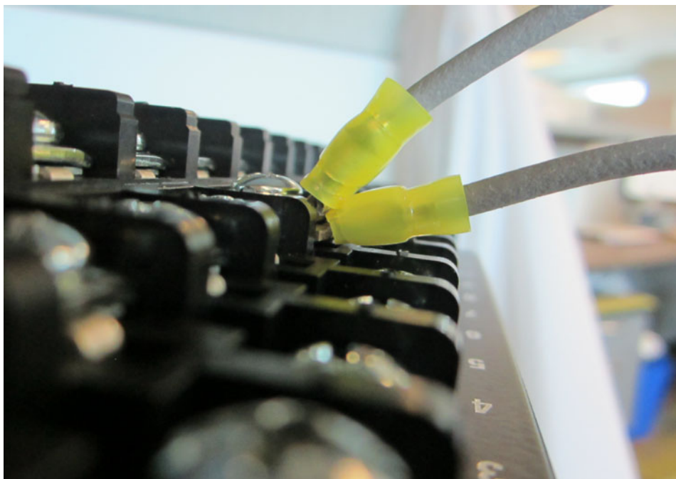
Figure 2-30: CORRECT INSTALLATION METHOD
