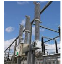
Live Tank circuit breaker up to 245 kV
