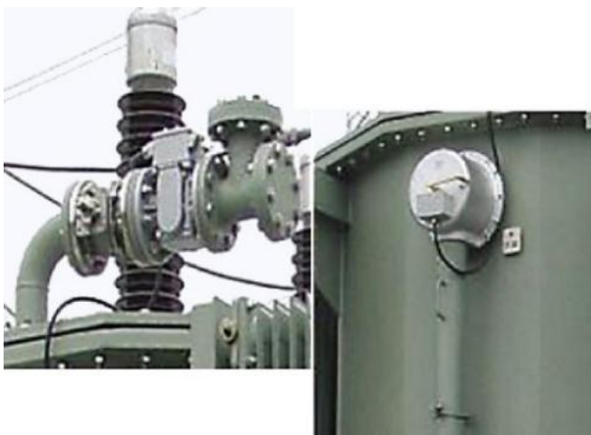
Fig. 3: Buchholz relay and pressure relief valve
