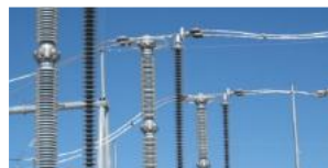
Instrument Transformers
