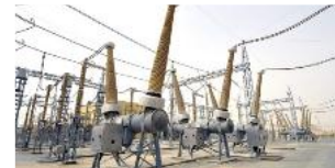
Circuit Breakers
