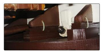
**Figure 6:** View of clamping brackets on LV side of one phase after the winding re-clamp. The photo shows how cable ties were used to secure blocks and shims.
