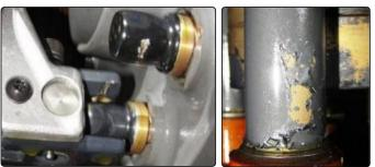
**Findings:** Silver sulphide on de-energized tap changer of a large 35 year old 330 kV/138 kV/11 kV auto-transformer.
