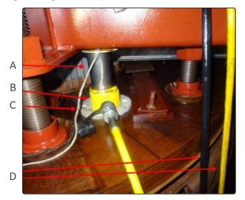
**Figure 5:** Example with one of the four hydraulic jacks in position between the clamping beam and the top winding platform, with load spreader to distribute the pressure. All four hydraulic lines were brought in through the HV turret.
