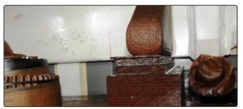
**Findings:** The clamping on one phase was found to be loose. The group of shims and thin block was so loose that it could be pulled out by hand.
