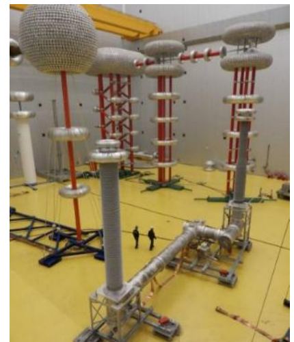
Voltage withstand and bus-charging current switching tests
