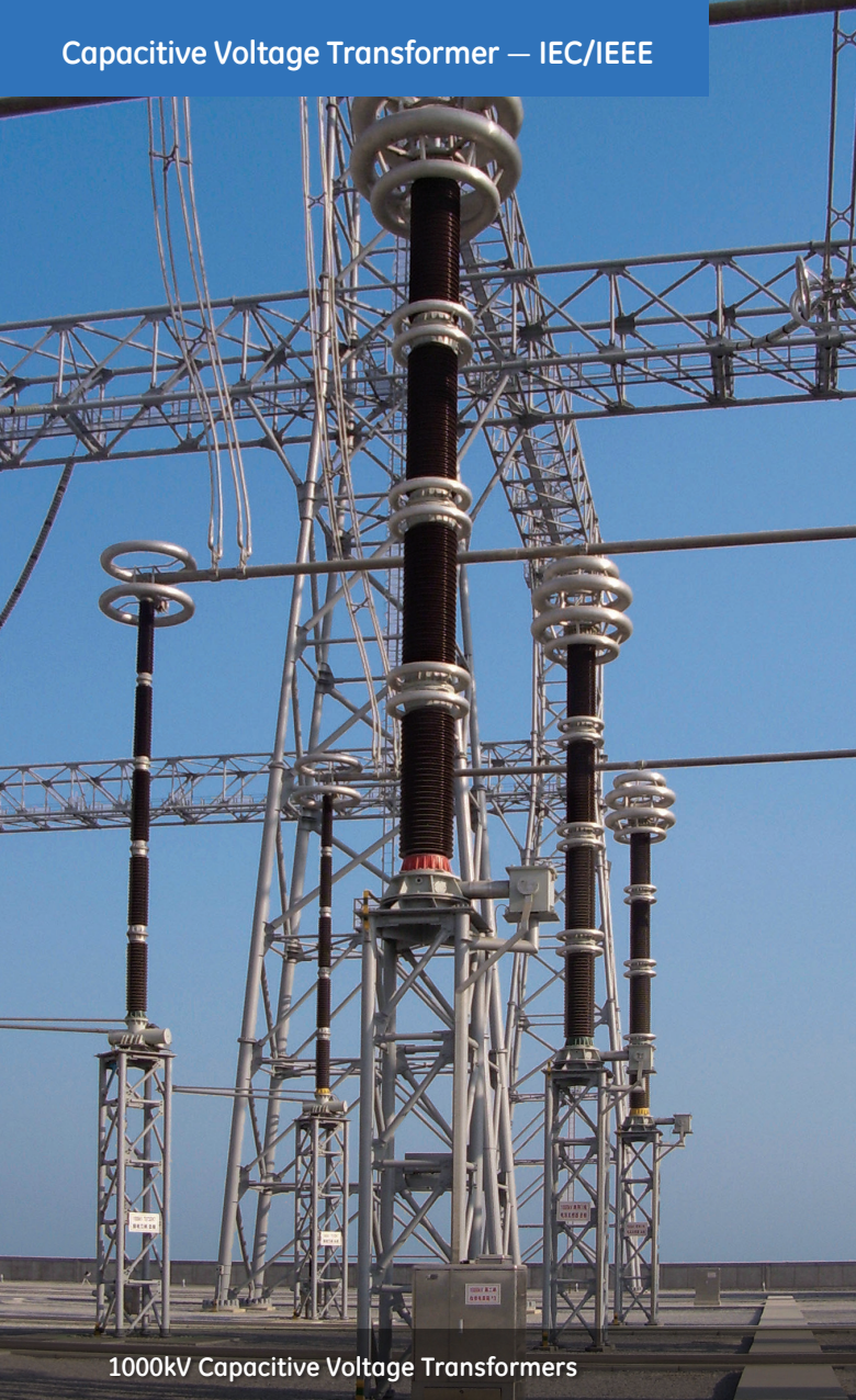
1000kV Capacitive Voltage Transformers
