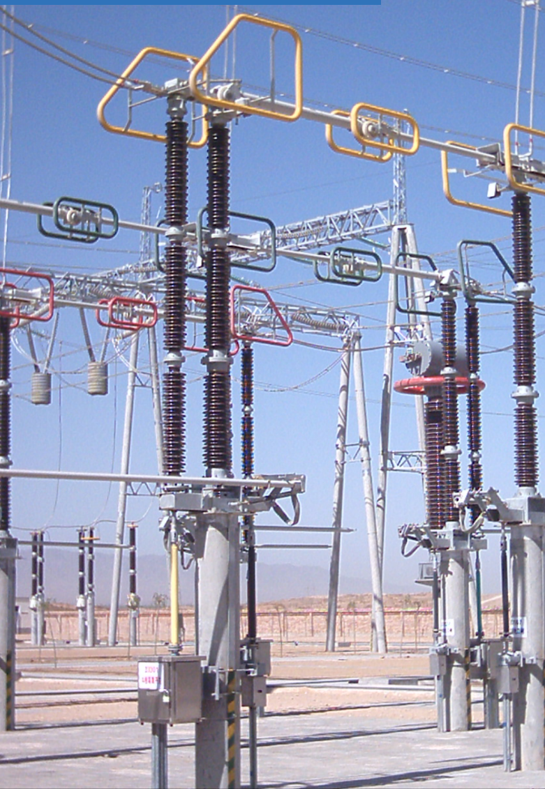
GW11-363kV Disconnect Switch
