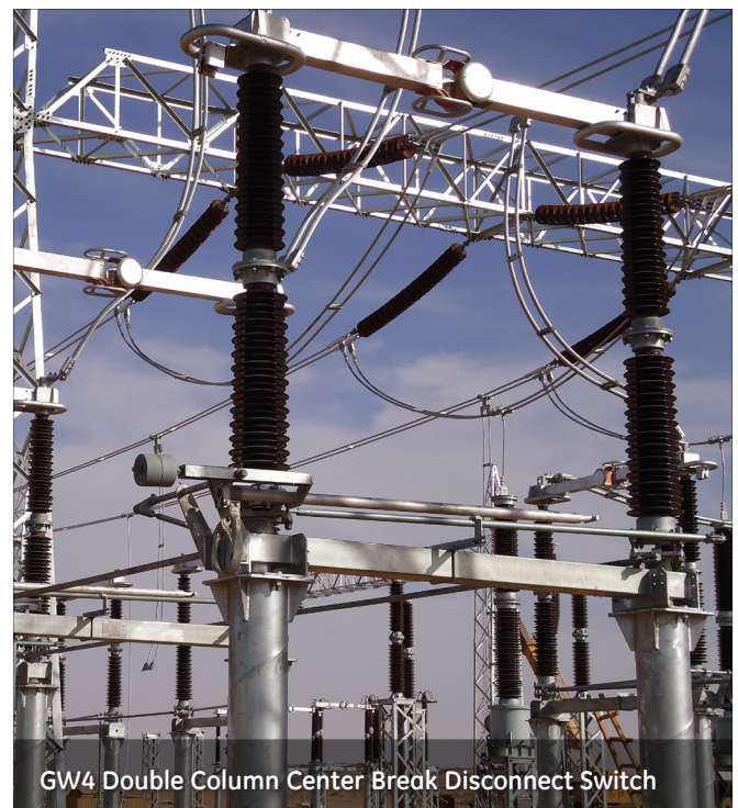
GW4 Double Column Center Break Disconnect Switch
