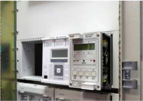
Withdraw the KCGG relay
