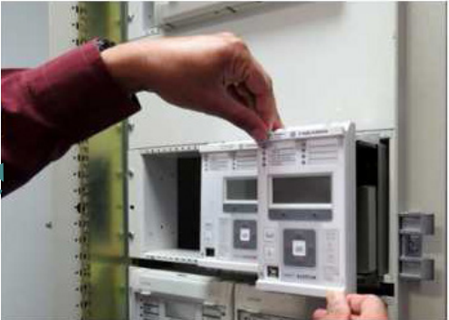
Replace with Agile P14N relay
