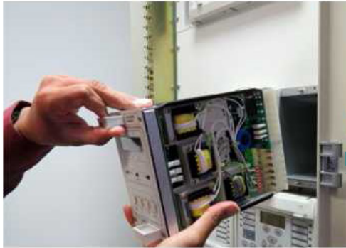
KCGG relay being taken out
