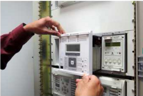
Replace with Agile P14D relay
