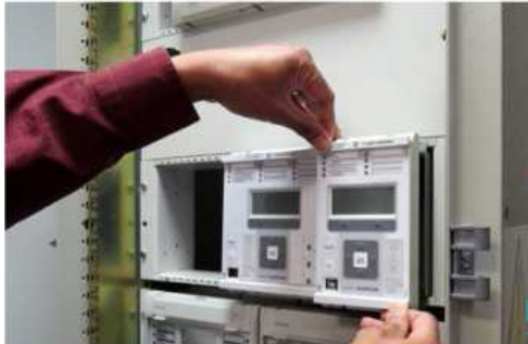
Old relays are replaced
