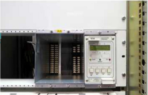
Withdraw the KCEG relay
