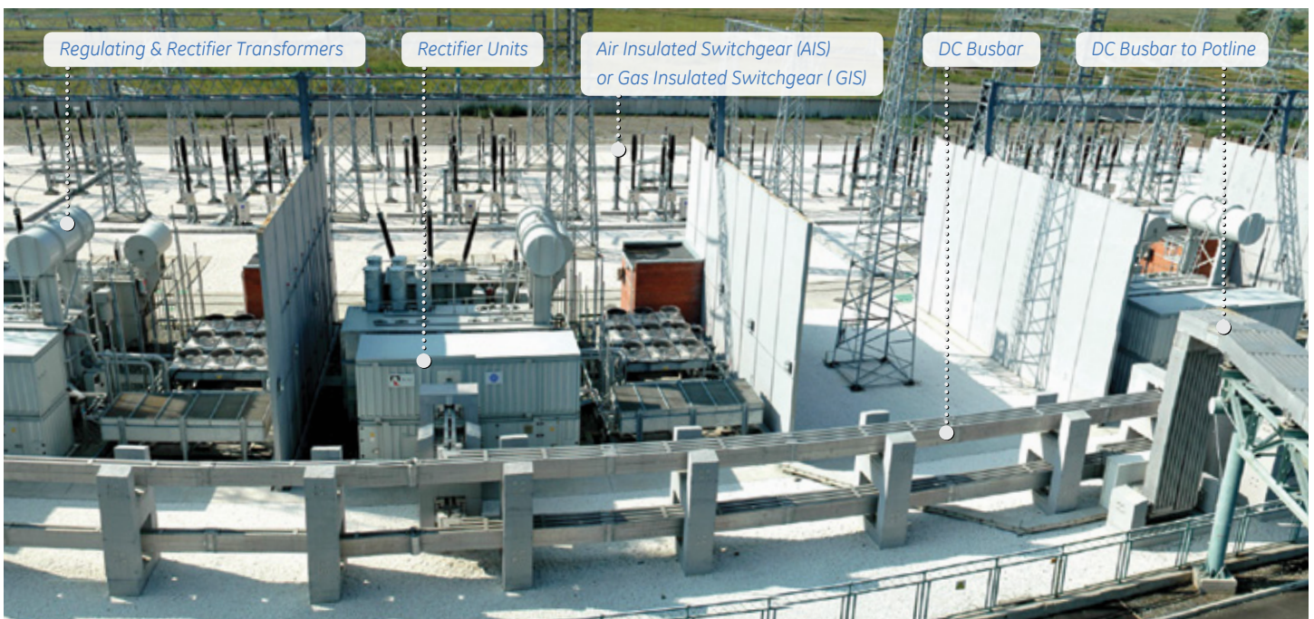
Typical DC System - Aluminium Smelter Conversion Substation
