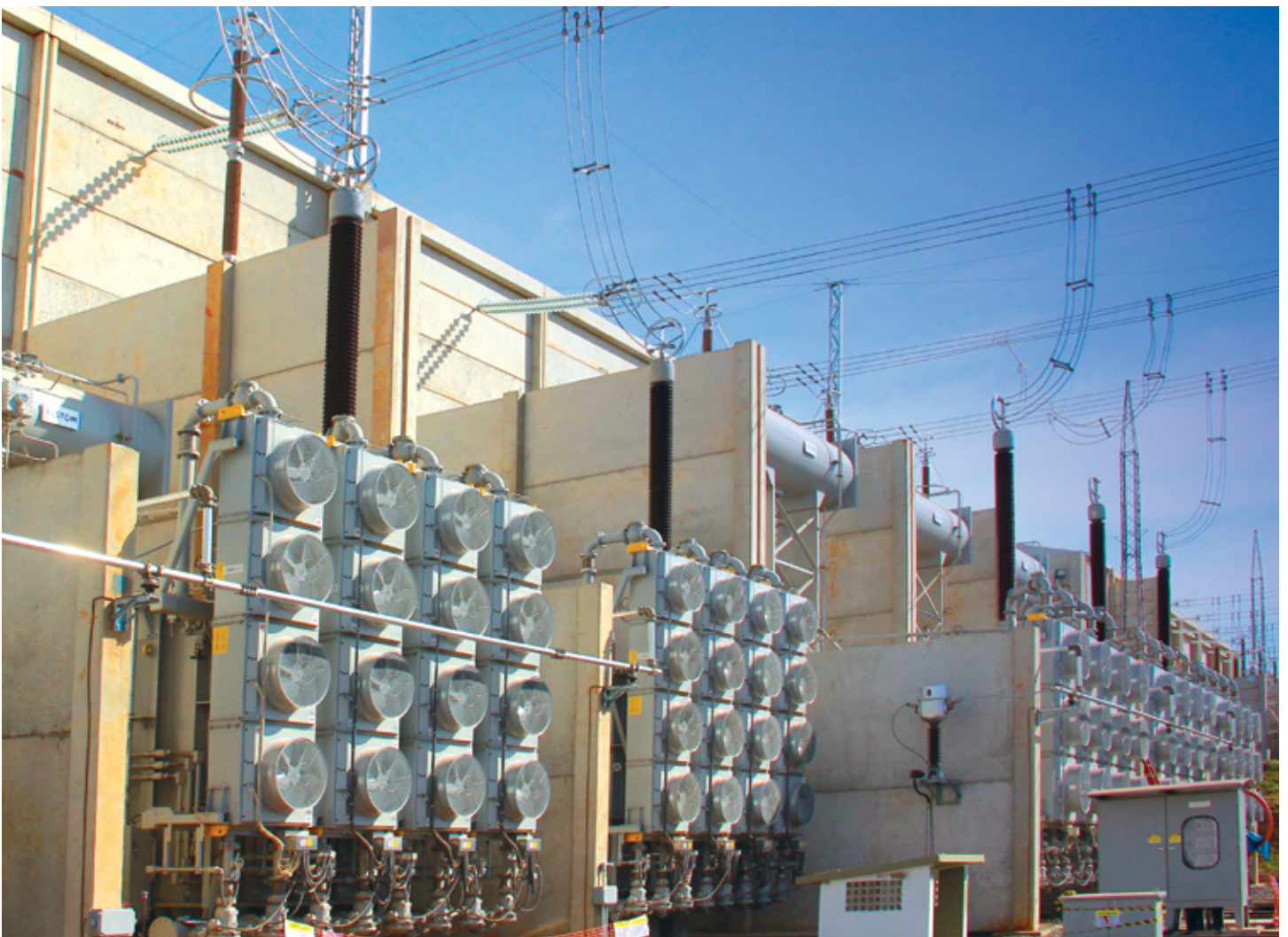
Converter Transformers
