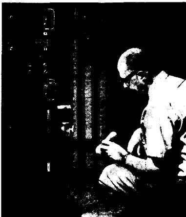
Fig. 1 INSPECTION BETWEEN PANELS need only be done at infrequent intervals since areas are protected from most nicks and scratches.
