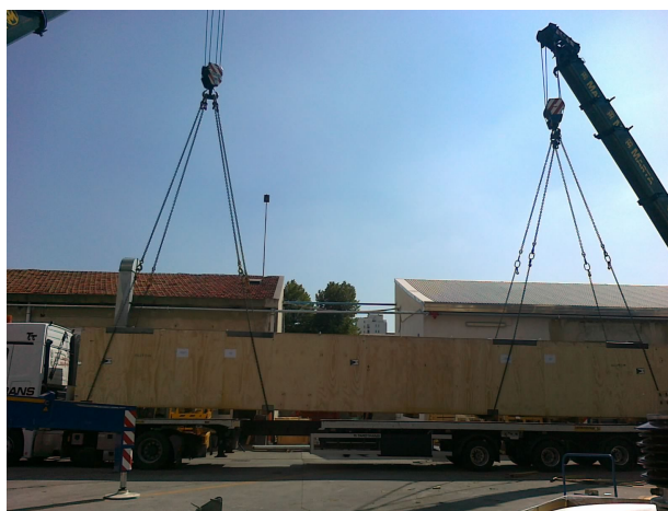
Figure 1 – Example of two crane lifting arrangement
