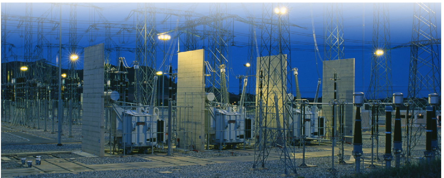
Single-phase autotransformers 500 MVA 765/400/20 kV in operation since the early 80's for EDELCA (Venezuela)
