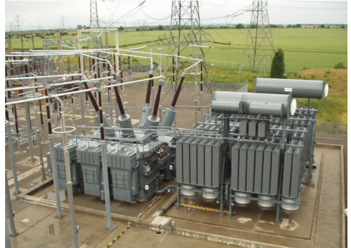
Quadrature Booster 2750 MVA 400/80 kV for National Grid Co. plc. High Marnham (UK)
