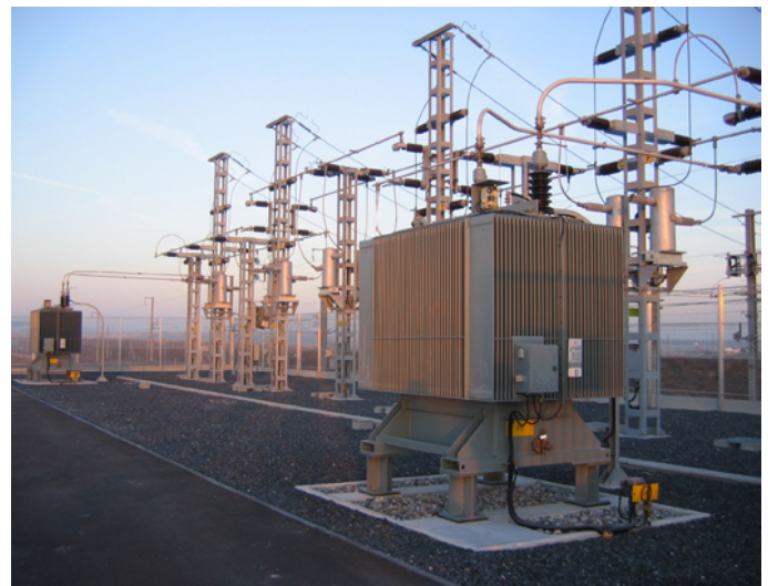
Autotransformers in SNCF railways (France)
