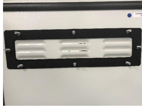
Figure B-8: Louvre gasket – tray removed
