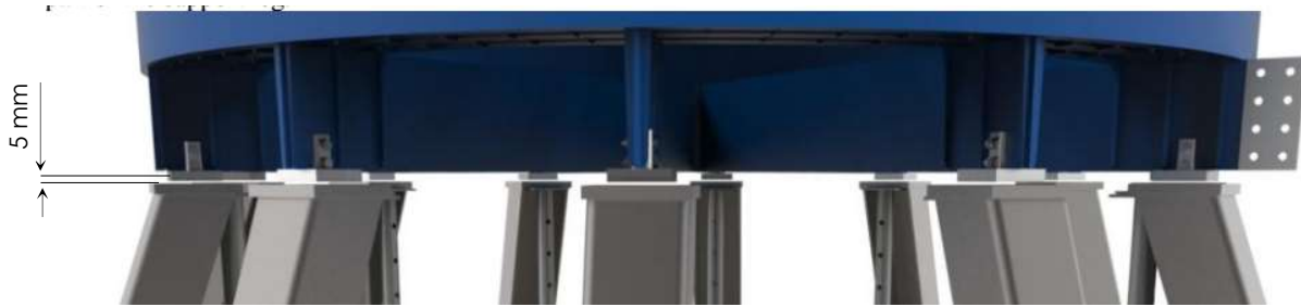
Figure 4: Clearance of 5 mm from the upper part of the supporting structure.
