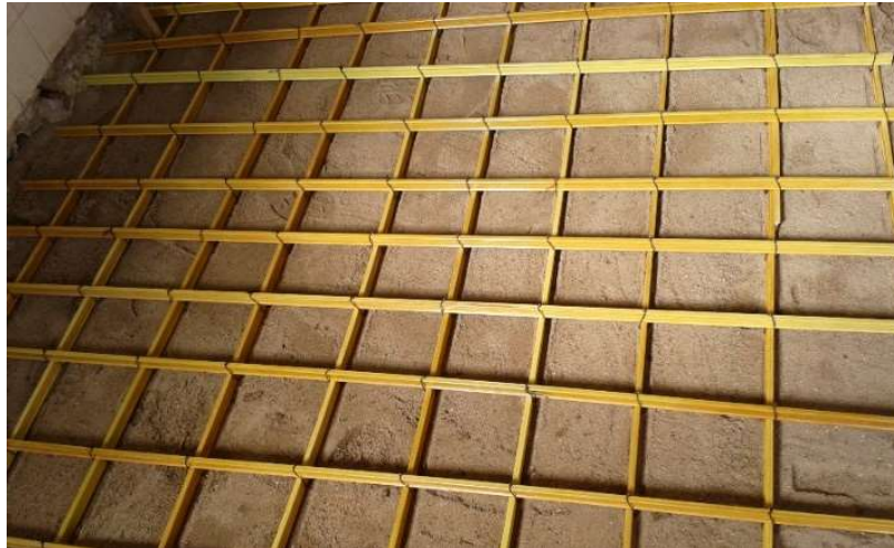
Figure 7: Foundation reinforcement using non-metallic (fiberglass) material.
