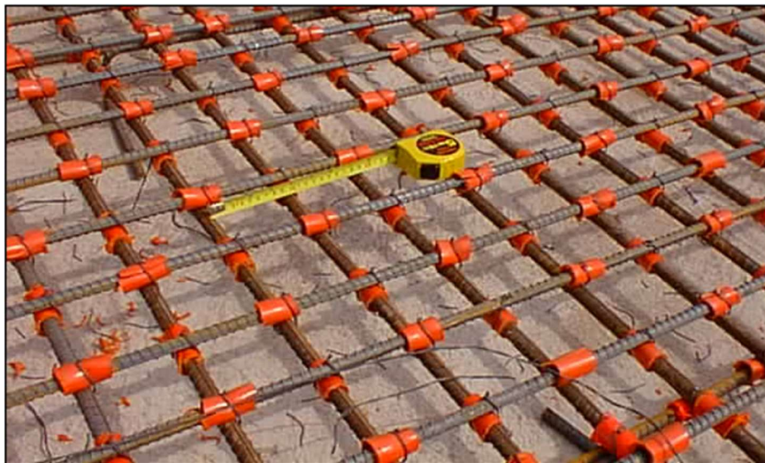
Figure 8: Magnetic insulation for foundation rebars.
