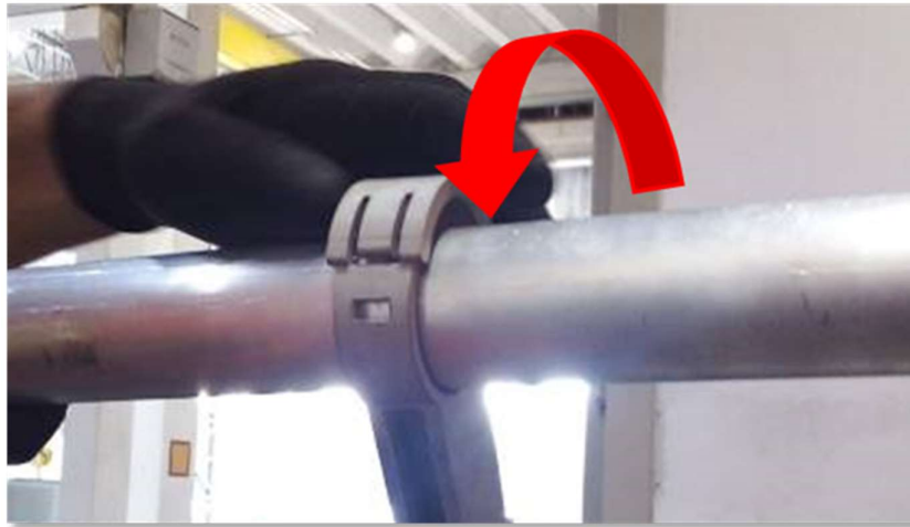
Figure 18: Lock cap detail.
