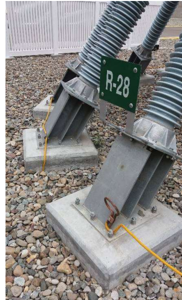
Figure 12: Earthing of base pedestals (Example with 12 points).
