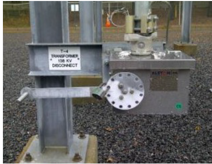
Disconnect switch manual mechanism
