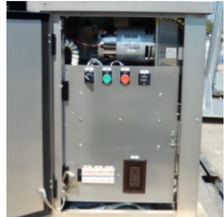
Disconnect switch motor operator
