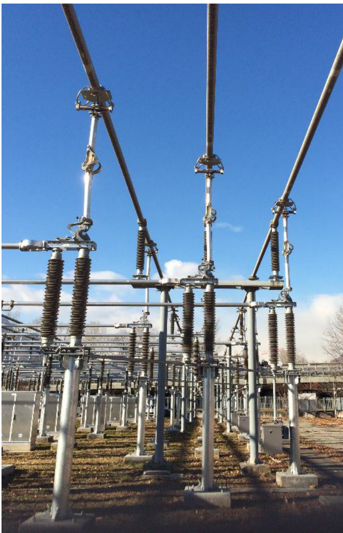
SPVL disconnecter type with DWatch mechanism installed
