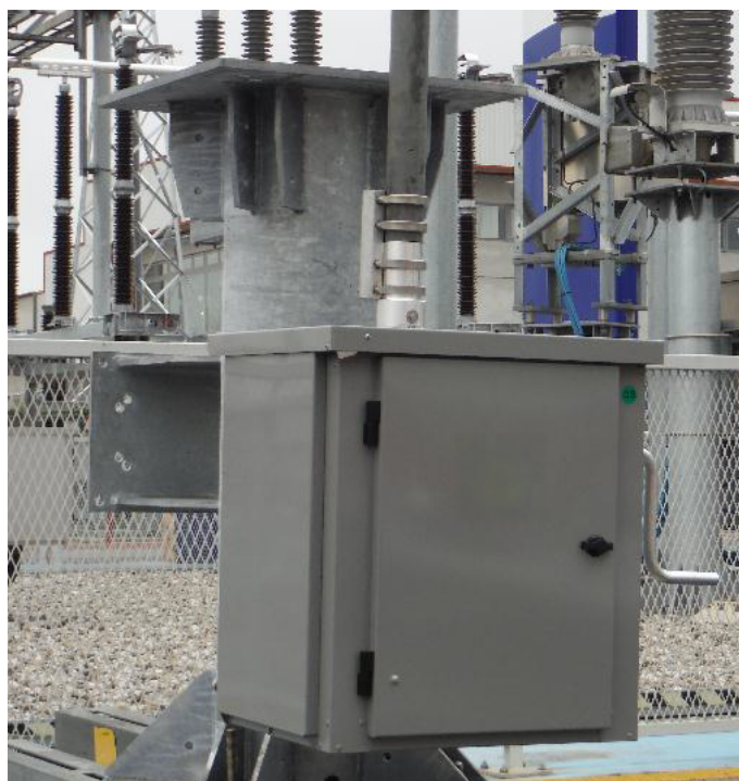
Typical installation of DWatch mechanism - external view
