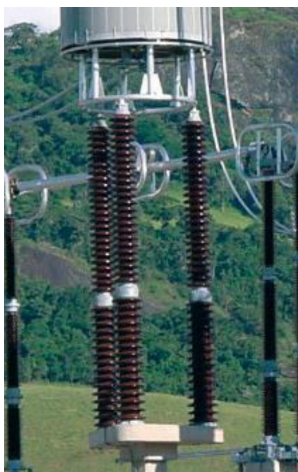
Vertical pedestal A line trap mounted on CCVT
