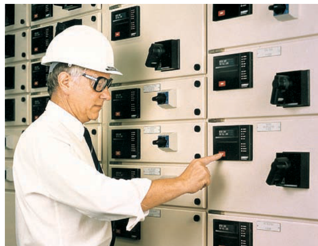
One MM2 is typically mounted in each starter of a motor control center.
