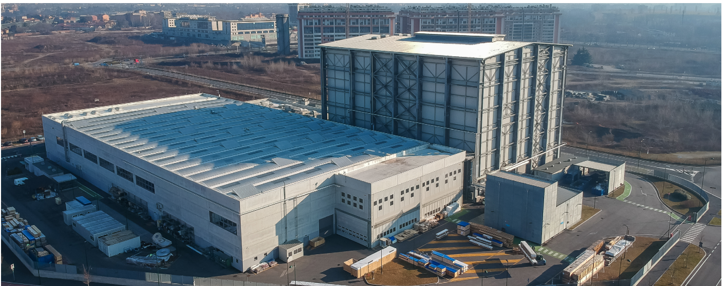
Manufacturing Site: Grid Solution, Sesto San Giovanni, Milan, Italy
