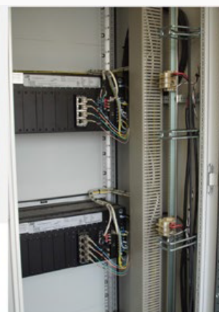
Simplified Fiber Optic Wiring of Protection Devices – Copper wires are replaced by a few fiber optic cables
