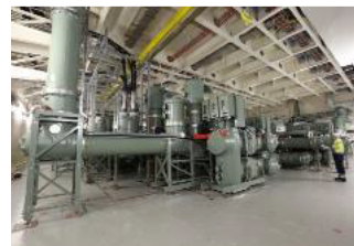
GIS Installed on the AC Substation
