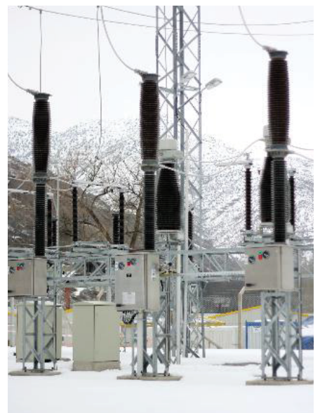
170 kV live-tank CB with single-pole operation
