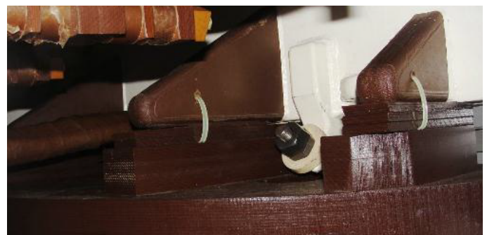
Figure 6: View of clamping brackets on LV side of one phase after the winding re-clamp. The photo shows how cable ties were used to secure blocks and shims.
