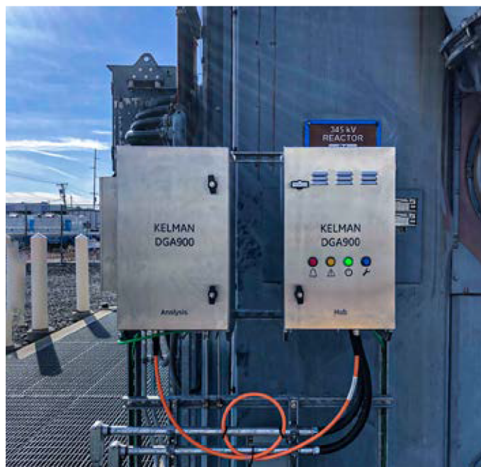
Kelman DGA 900 installed on NYPA transformer
