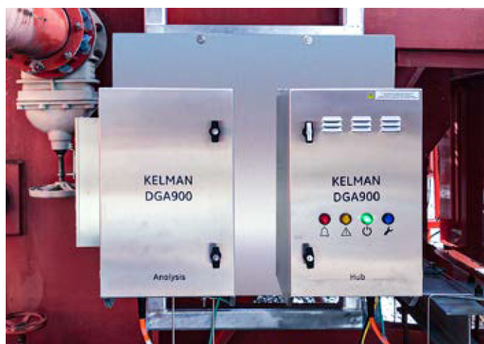
Kelman DGA 900 installed on NYPA transformer
