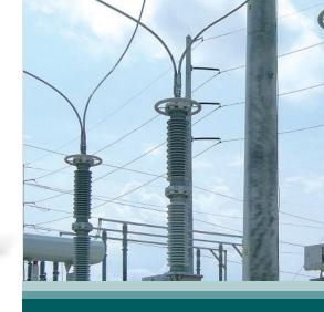
In high and extra high voltage transmission systems, capacitor voltage transformers (CVTs) are used to provide potential outputs to metering instruments and protective relays. In addition, when equipped with carrier accessories, CVTs can be used for power line carrier (PLC) coupling.
