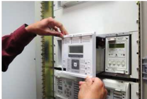
Replace with Agile P14D relay
