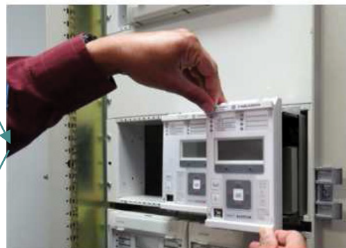
Replace with Agile P14N relay
