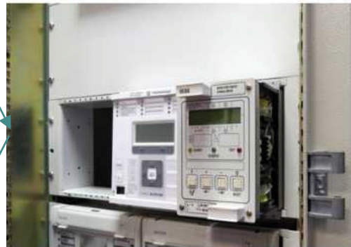
Withdraw the KCGG relay
