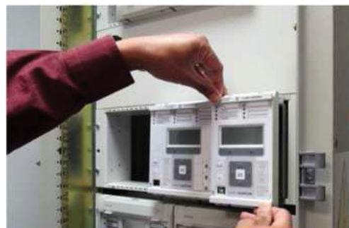
Old relays are replaced
