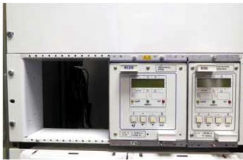
Typical relay panel with KCEG and KCGG Relays
