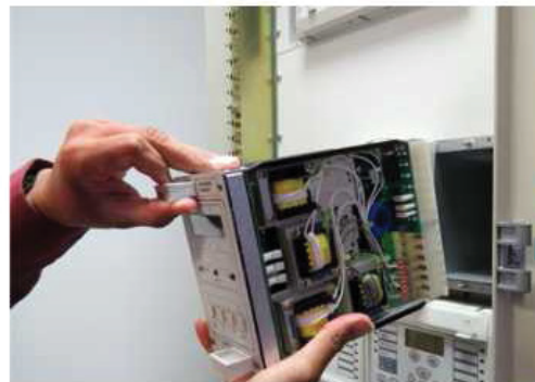
KCGG relay being taken out
